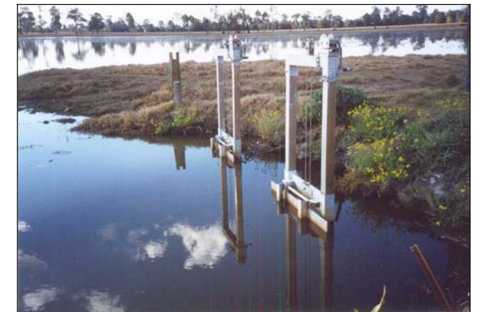
Secondary water control structure holding water on wetland areas
