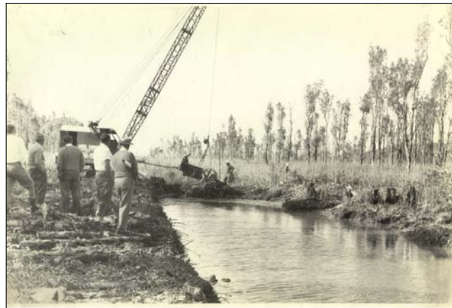
Dragline used to construct drain at Killick Creek, Kempsey NSW
