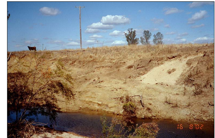
Erosion of a streambank in Myrtle Creek, Casino. The extent of erosion has been exasperated by cattle accessing the stream for water (photo G. Owers)
